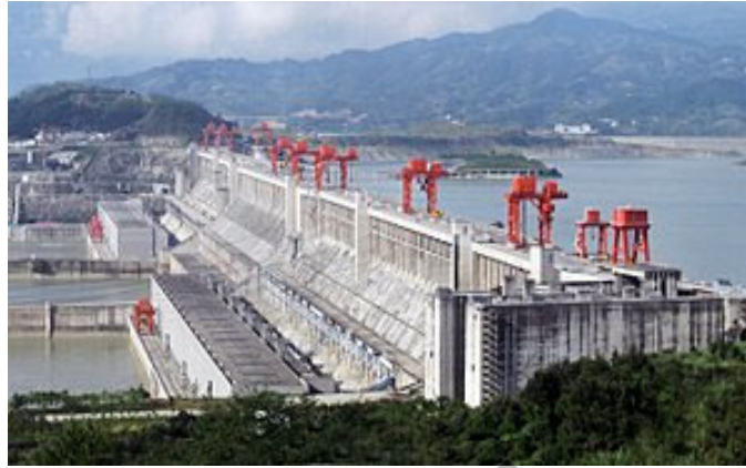
Fig. 4.9. Aboveground hydro power station
