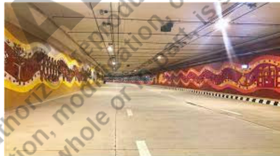
Fig. 4.10. Tunnel at Pragati Maidan, India
