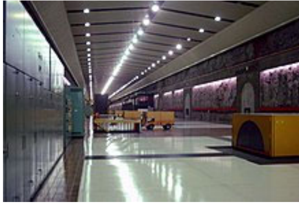
Fig. 4.8. Underground hydro power station
